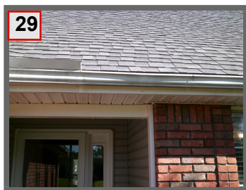
Shingles showing signs of weathering & age.
